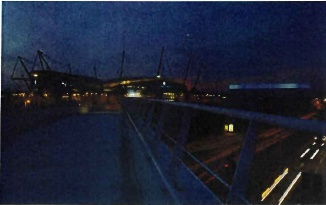
View 3 – View from eastern end of pedestrian footbridge leading to Commonwealth Way, Etihad Stadium (night-time)
