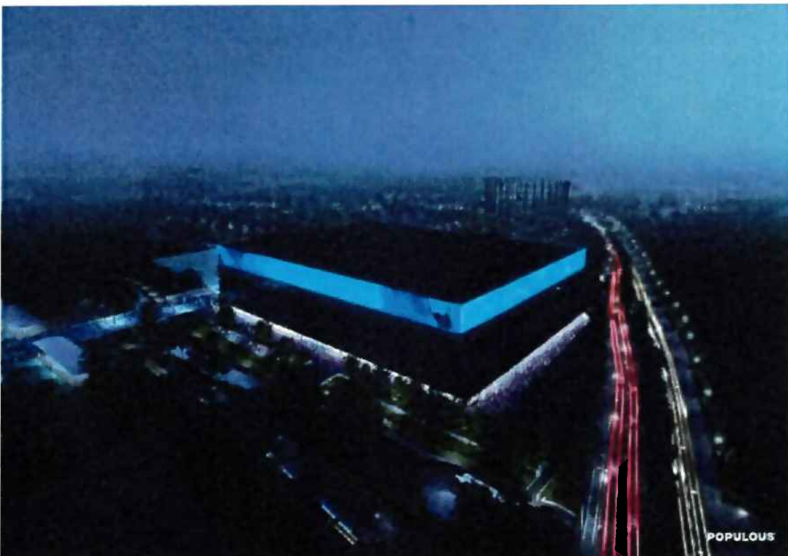
Aerial view of the arena with its high gloss black facade, lighting and LED screens together with soft landscaping
